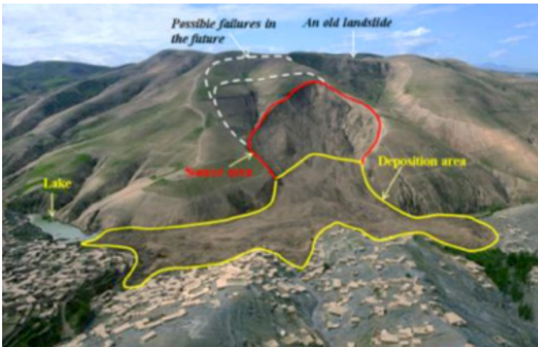
Image 11 An overview picture. There is an old landslide (with unknown age) next to the recent one, indicating that this region is prone to landslide hazards. The white dashed lines show the possible failure scarps in the future (Source and Copyright: The Atlantic)
