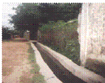
Figure 11: Constructed Urban drain
