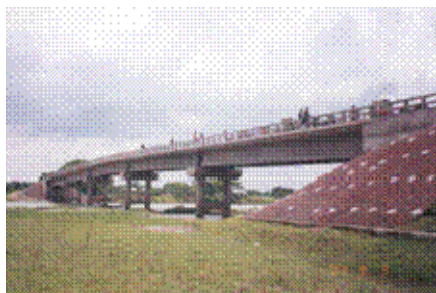
Figure 7: Span increased and approach strengthen
