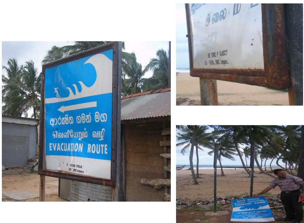
Figure 4: Corrosion and damaging the sign boards
