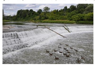
Figure 28 Flood Mitigation Dam to reduce downstream water velocity (Source: https://www.bestnetfax.com/wp-content/uploads/2018/10/flood-control-wikipedia-how-do-floods-form.jpg)
