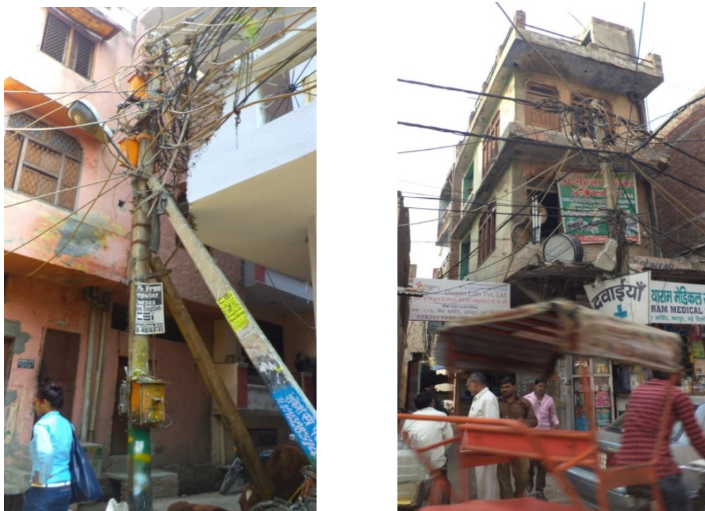
Fig.8 Illegal tapping of electricity, a common sight in urban villages of Delhi
