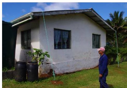
Figure 3: A house with the roof anchoring system.
