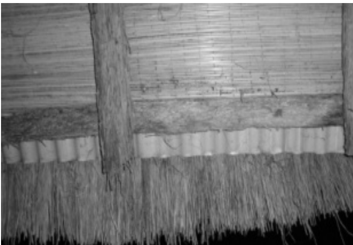
Figure 2. A composed covering of zinc and straw, combining the durability and waterproofing properties of the zinc (above) with the insulation qualities of the straw (below) is the best practice recommended for tropical conditions. Credits: The authors
