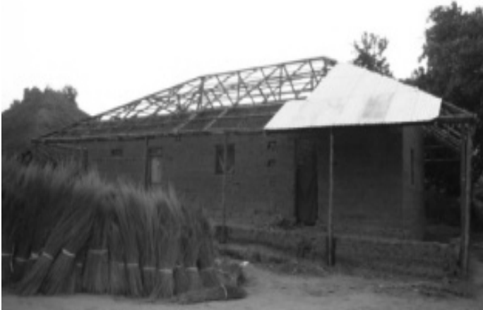
Figure 1. Vernacular houses in Guiné-Bissau usually built with rammed earth or adobe walls and straw fiber roofs (above), recently replaced by zinc (below). Credits: The authors
