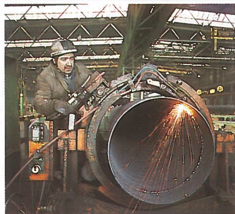
Válcovny trub Chomutov - manufacturing of one-piece-pipes, one of the final operations
